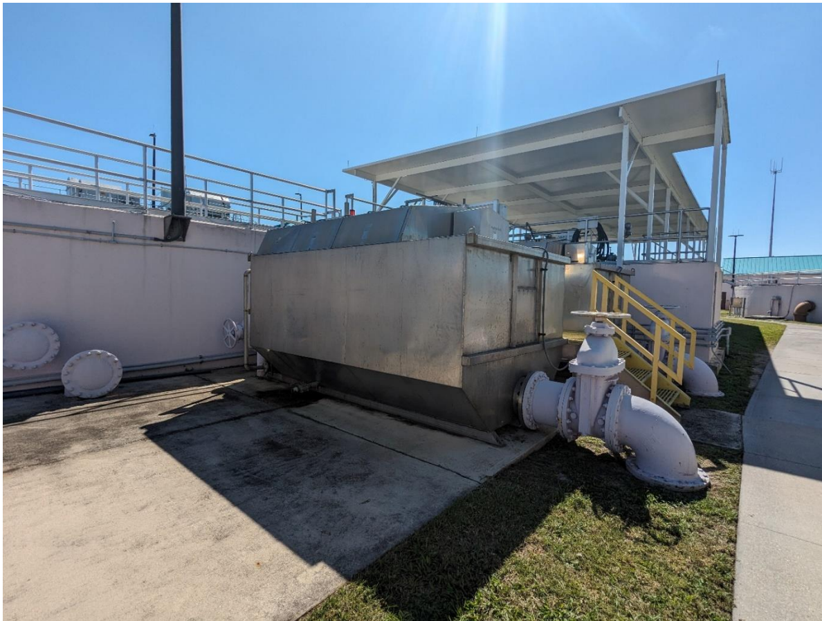
FIGURE 4-35: WRF DISC FILTERS
