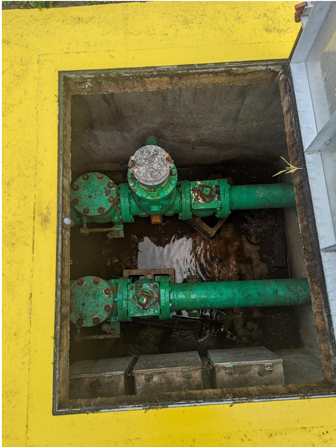
FIGURE 4-4: LIFT STATION 3 VALVE VAULT
