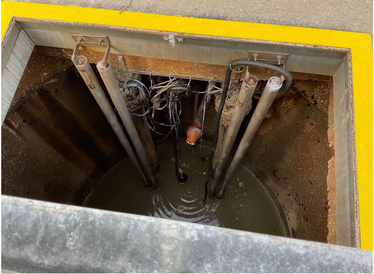
FIGURE 4-17: LIFT STATION 15 WET WELL
