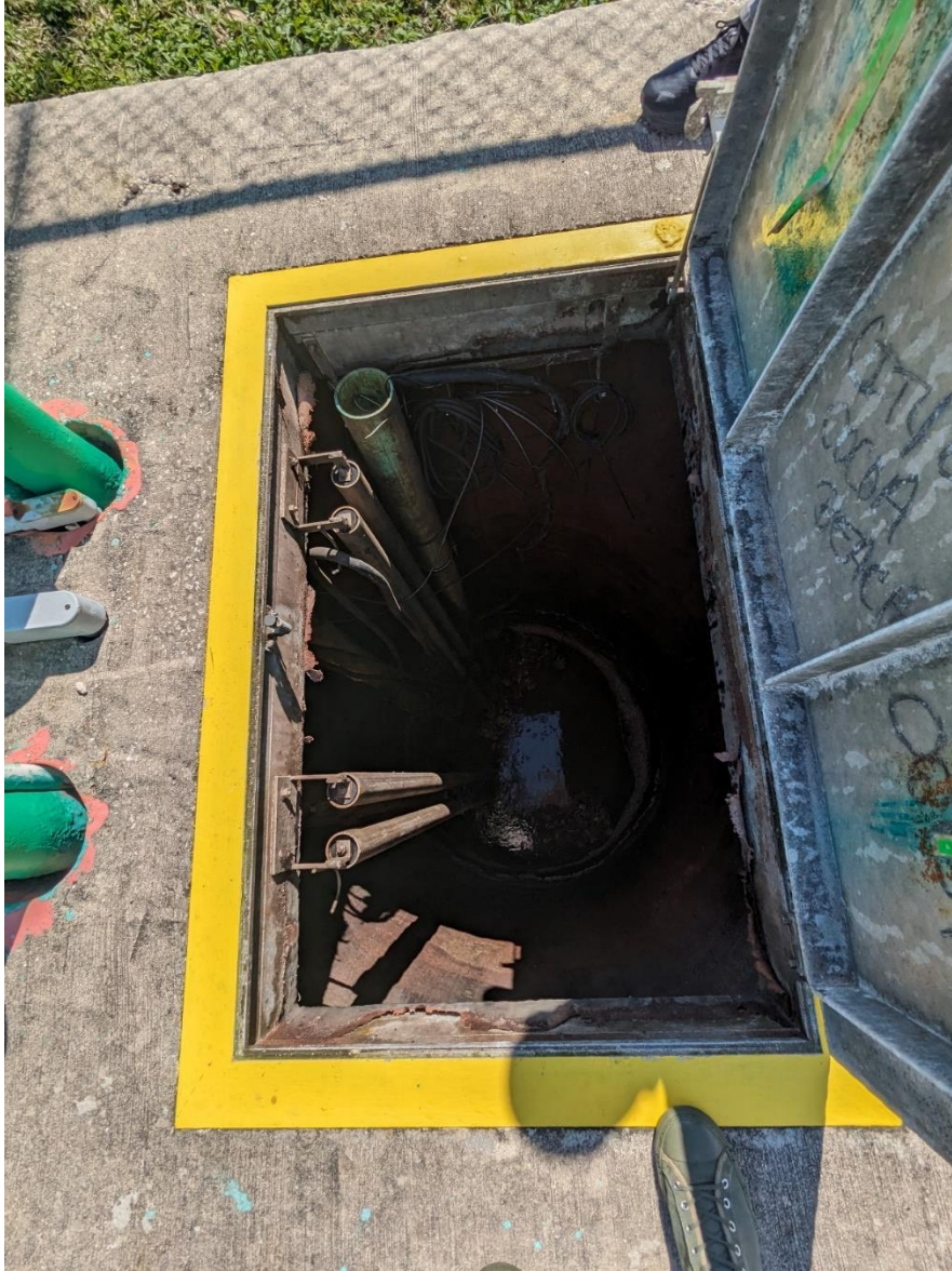
FIGURE 4-11: LIFT STATION 8 WET WELL
