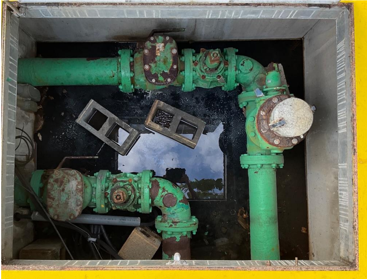
FIGURE 4-18: LIFT STATION 15 VALVE VAULT
