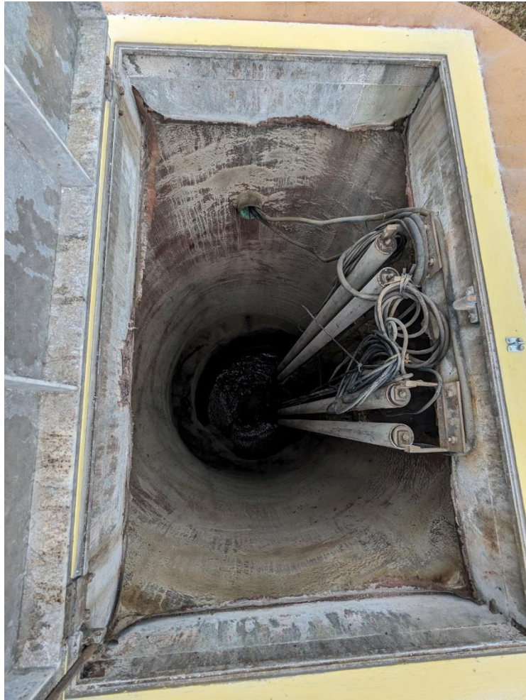
FIGURE 4-14: LIFT STATION 10 WET WELL
