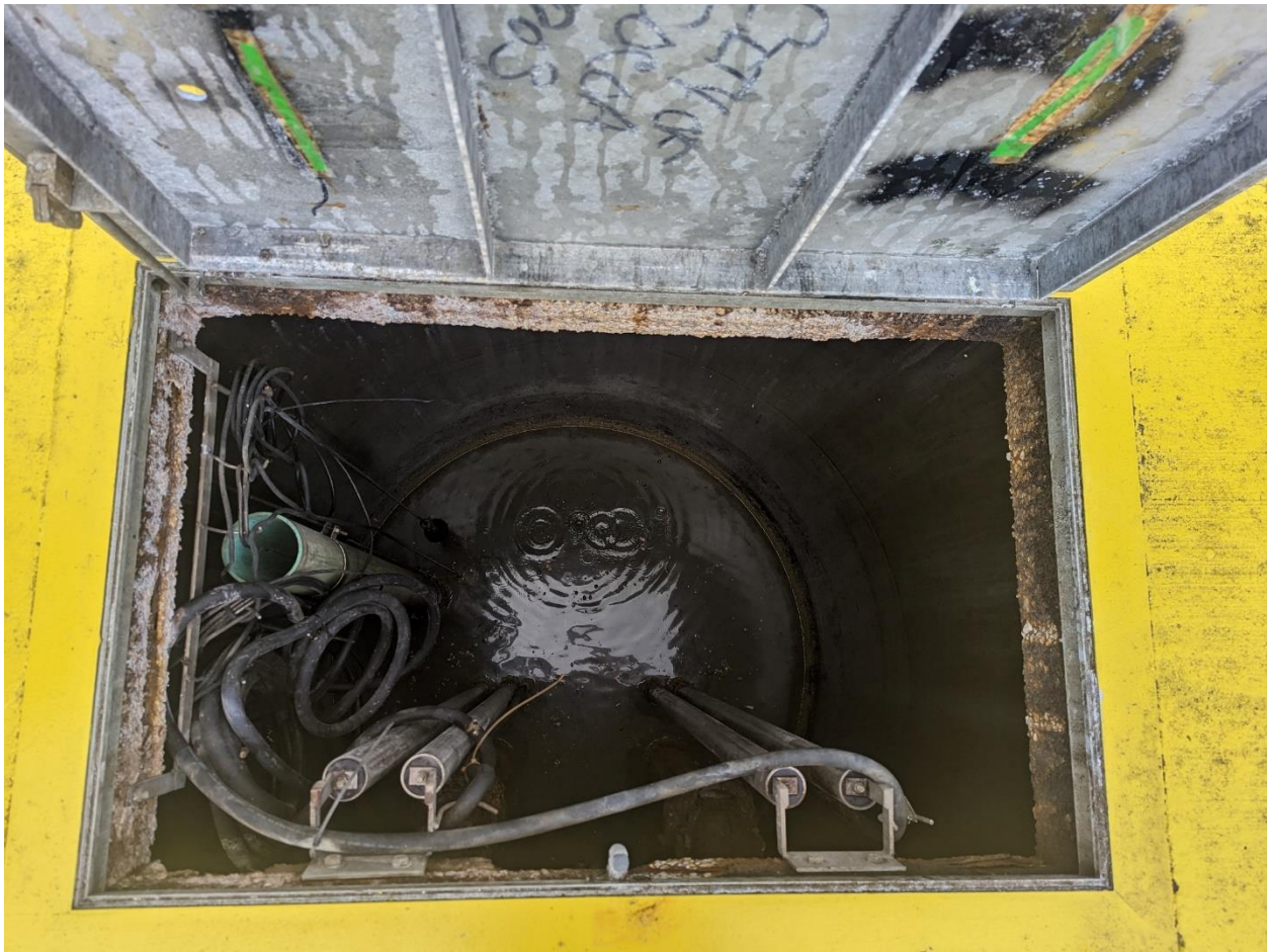
FIGURE 4-3: LIFT STATION 3 WET WELL
