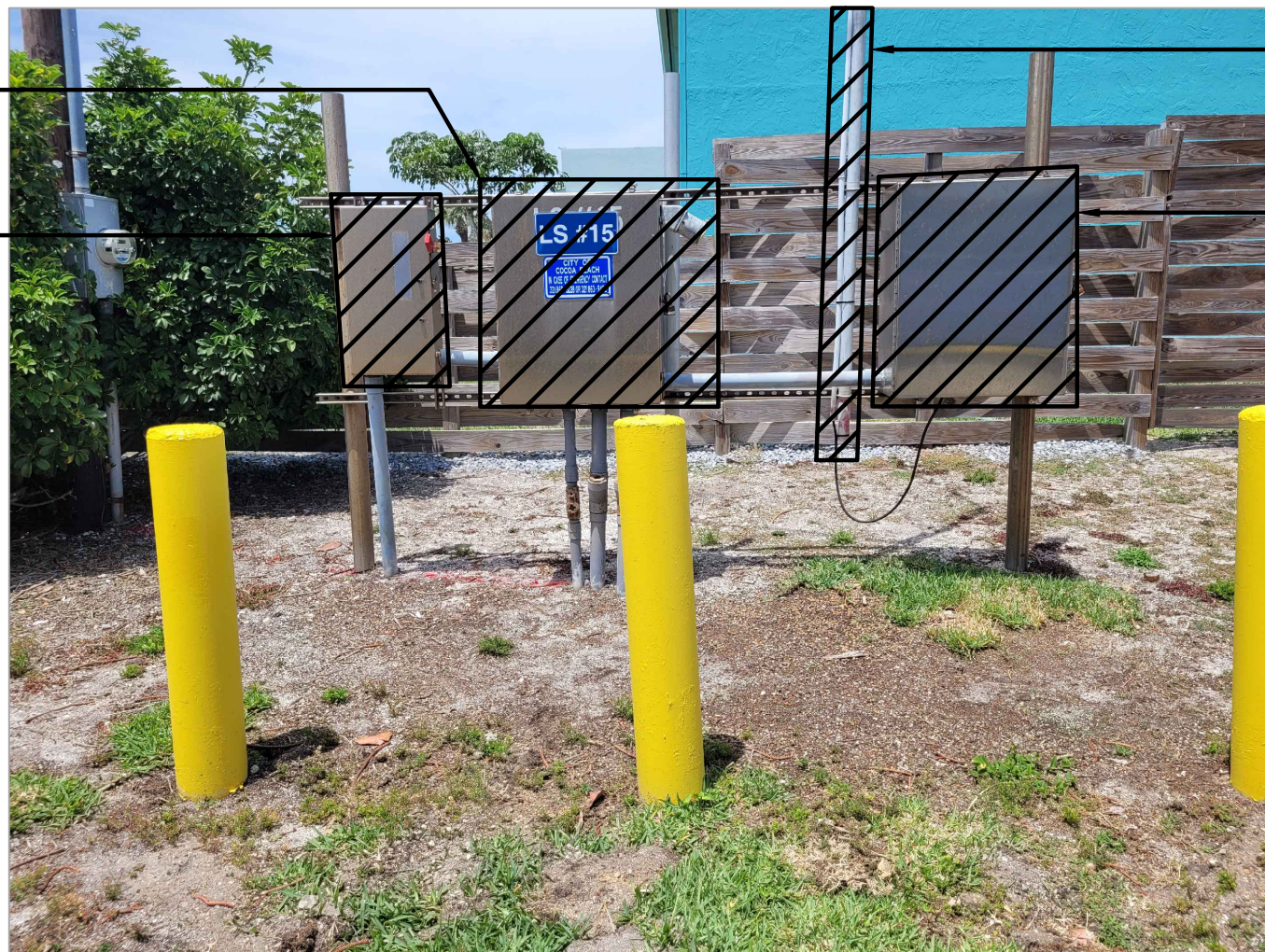
ELECTRICAL DEMOLITION PICTURE DETAIL 2
